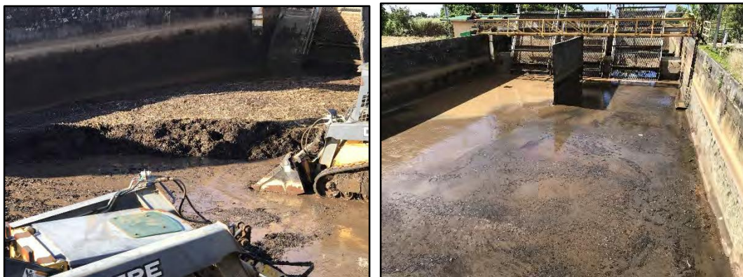
Wailoa Ditch cleanout – before and after
